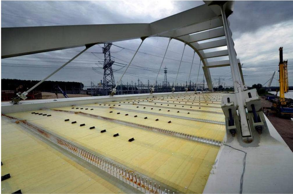
*Figure 1 Bridge with composite sandwich panels prior to casting concrete.*
